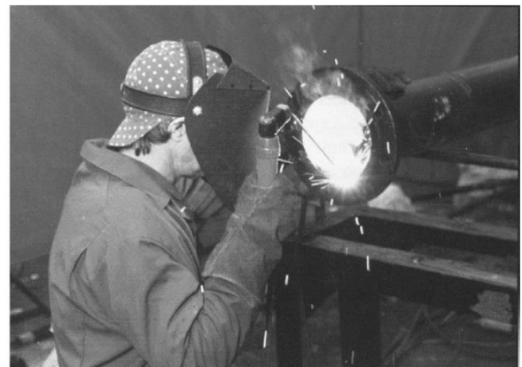
Fig. 8. Welder with appropriate personal protective equipment (NRPB 2002).
